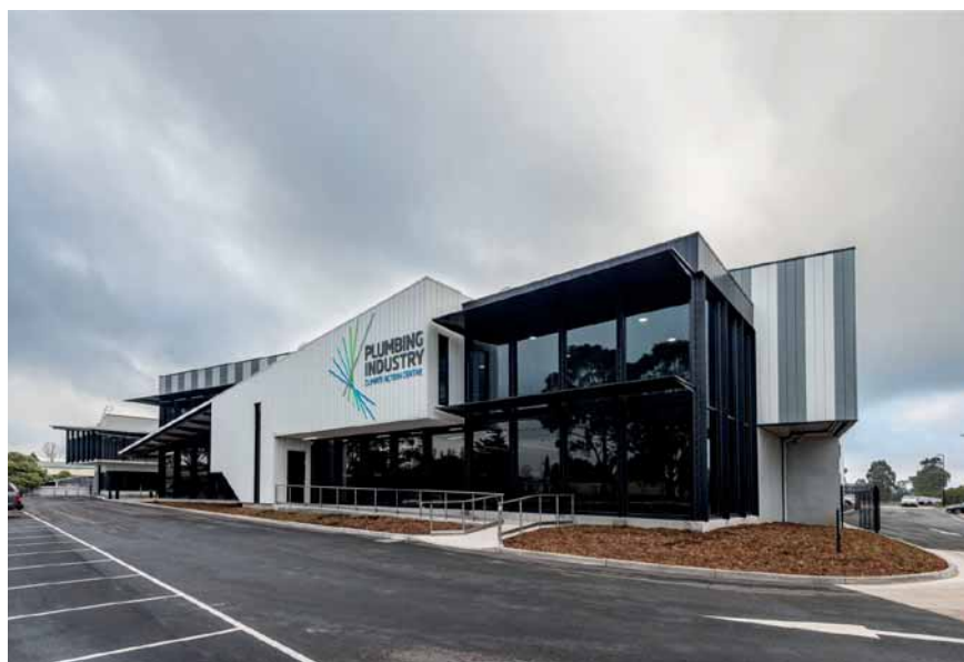
The Plumbing Industry Climate Action Centre (PICAC) is a center of excellence for learning and education for the plumbing industry.
