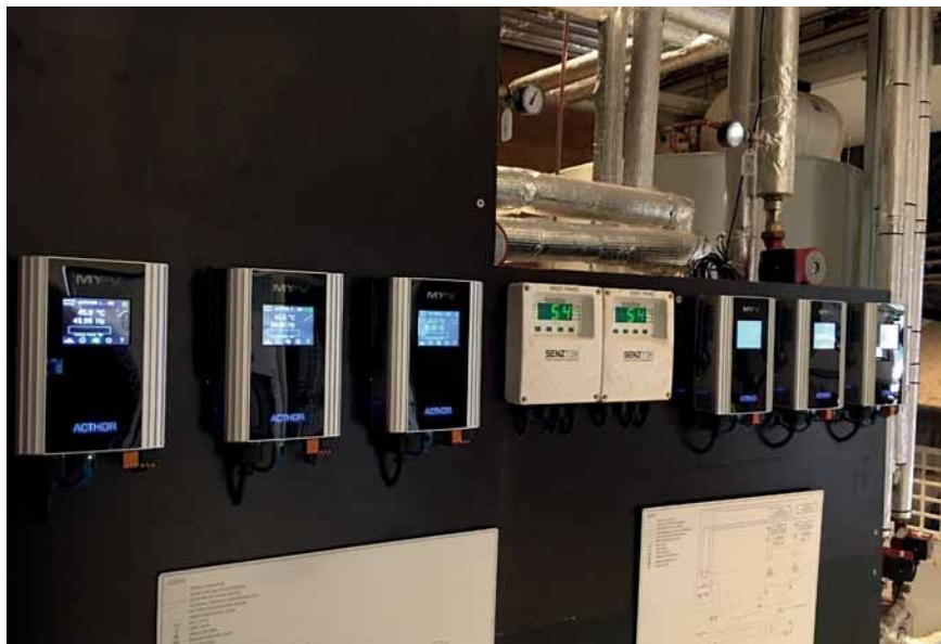
The AC·THOR can record data such as meter values and temperatures for current year, month or day that can be read off at any time.
